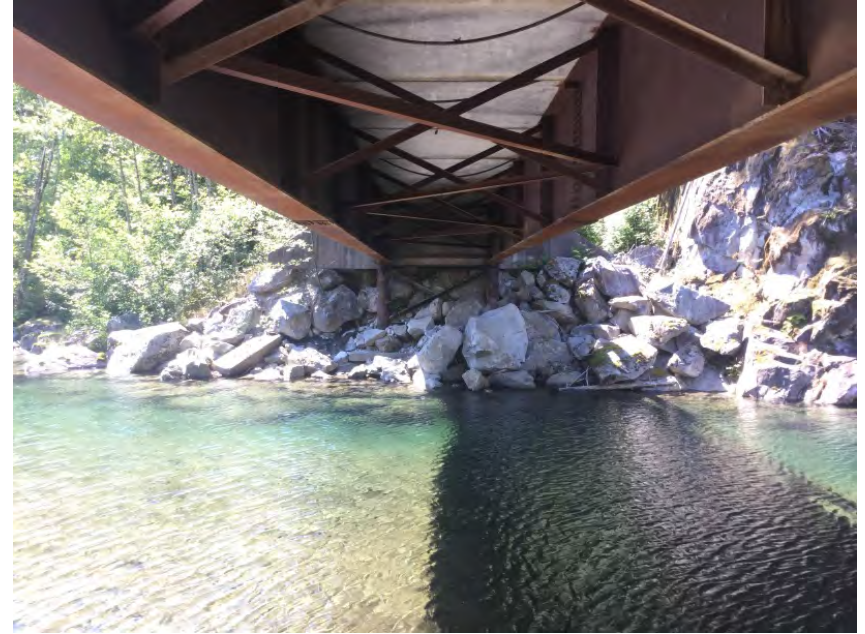
Right Bank Abutment
