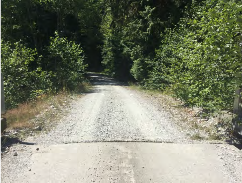
Right Approach Facing Away From Bridge
