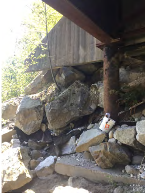
Right Abutment Downstream Corner
