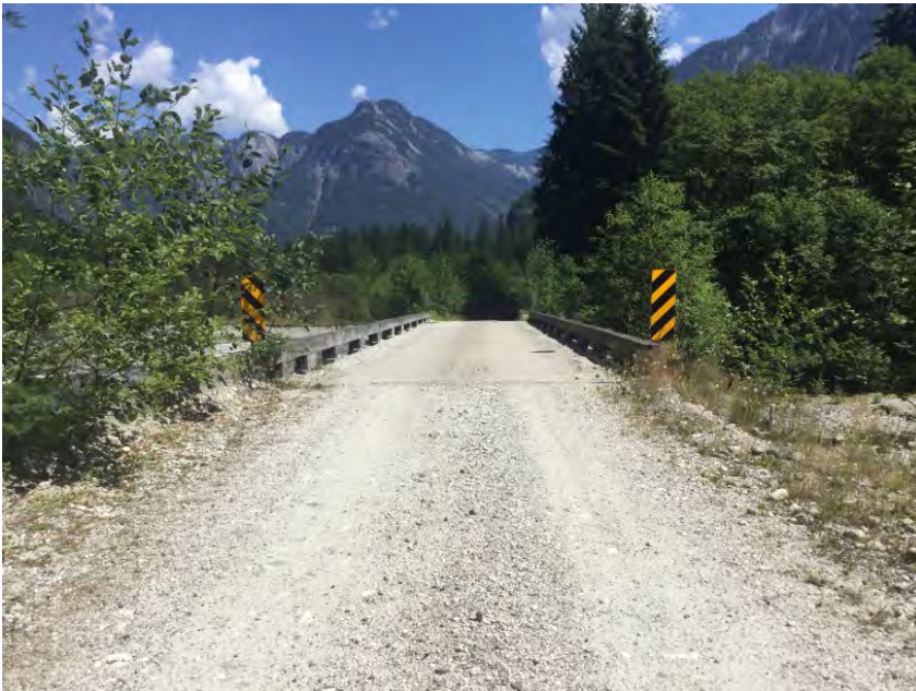
Right Approach Facing Bridge
