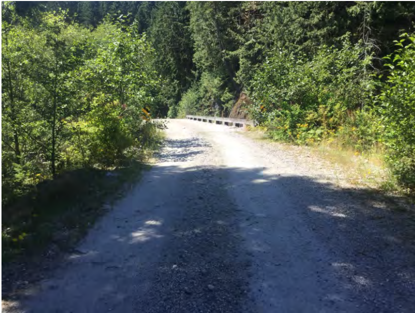
Left Approach Facing Bridge
