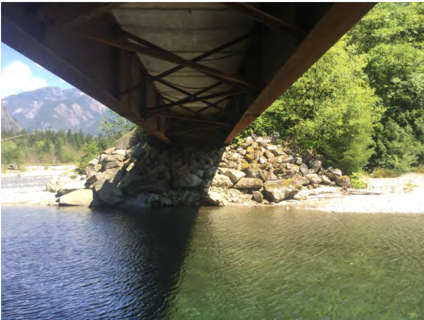
Left Bank Abutment
