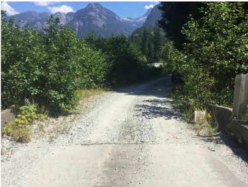
Left Approach Facing Away From Bridge
